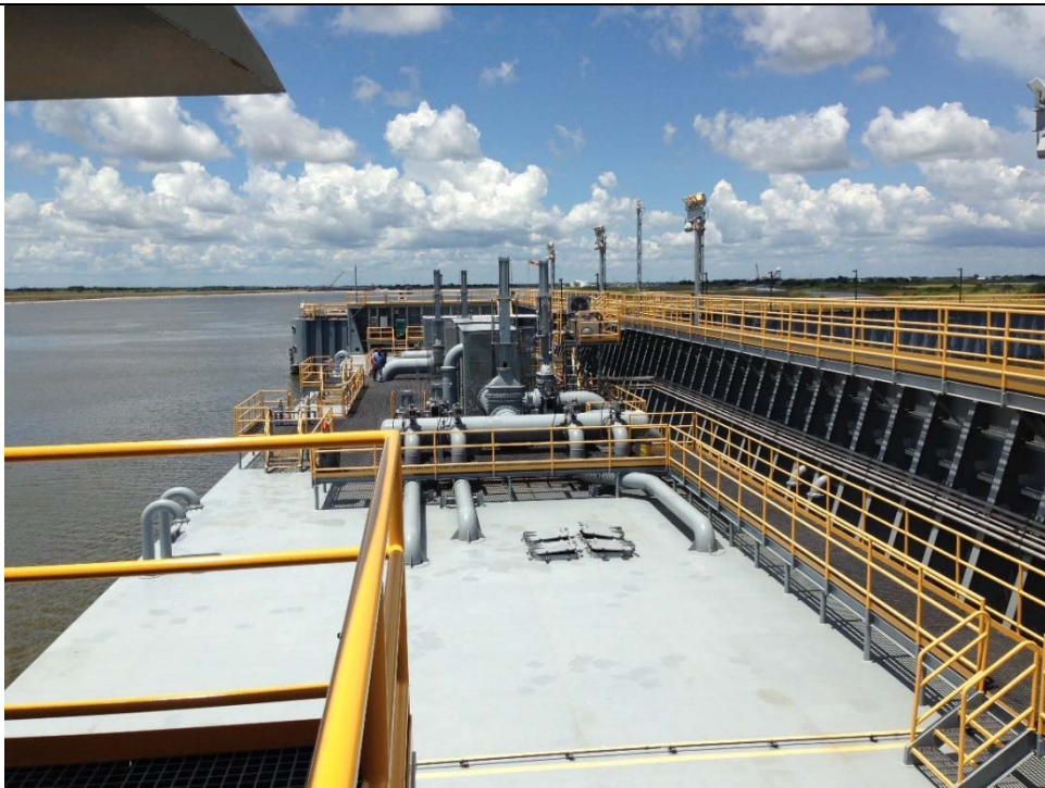
Picture 2: Bubba Dove Barge Gate, Houma Navigation Canal. The steel barge gate is 250-foot wide approx. 42 feet high. Design by CB&I (the former IHNC Shaw team).
