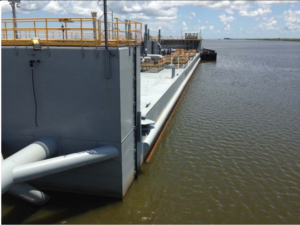
Picture 1: Bubba Dove Barge Gate, Houma Navigation Canal. The steel barge gate is 250-foot wide approx. 42 feet high. Design by CB&I (the former IHNC Shaw team).
